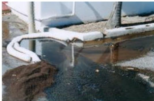
*Absorbent booms preventing spill entering a drain*
