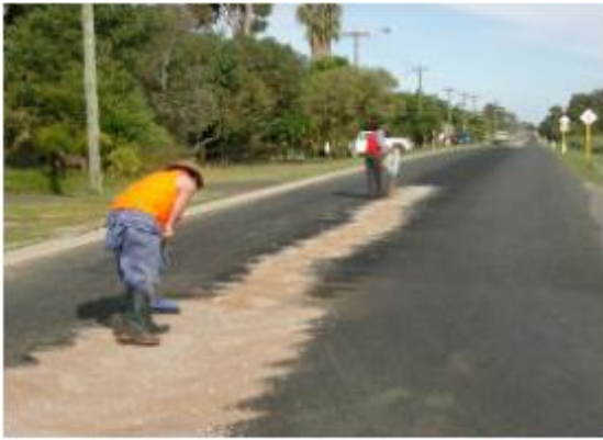
Prosorb Plus used to cover and absorb spill
