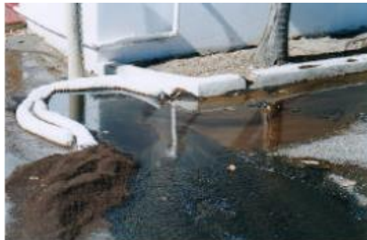
Absorbent booms preventing spill entering a drain
